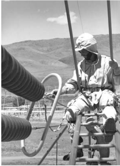
Figure 10-9. Bare-hand, live-line maintenance.
