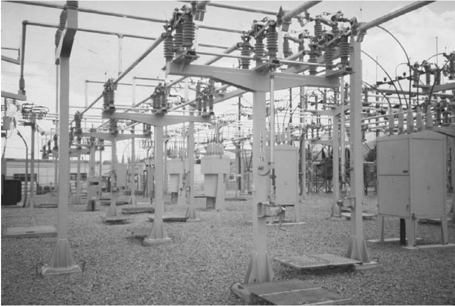
Figure 4-38. Examples of a typical electrical bus.
