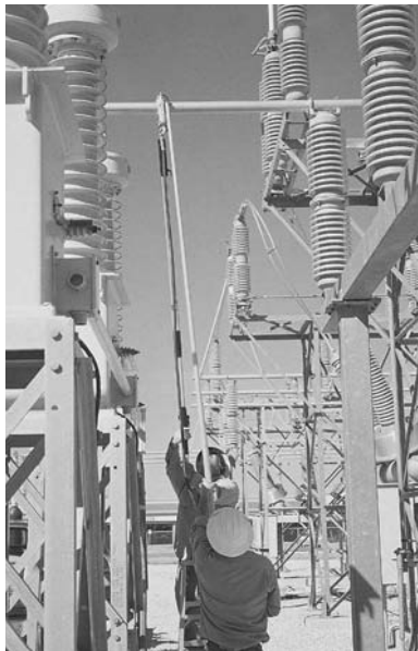
Figure 10-8. Live maintenance on transmission lines.
