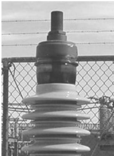
Figure 4-7. Bushing oil level gauge.
